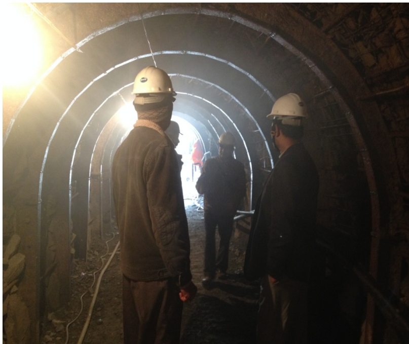
Figure 2: Test Adit Tunnel
