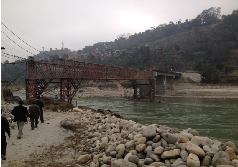
Figure 1: Bridge Under Construction
